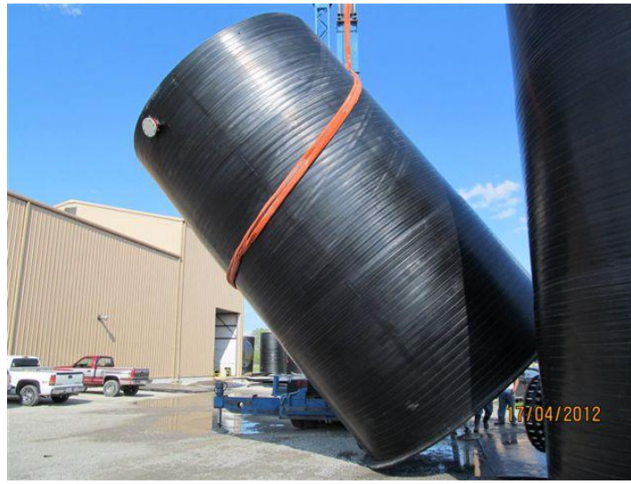
20' tall tank lifted with endless nylon sling at 2/3rds height.
