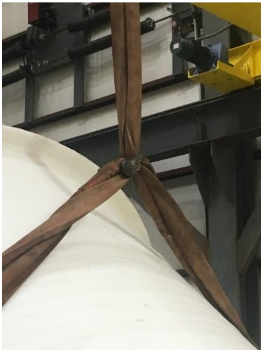
Picture 1: Nylon strap goes through metal choke clevis for tank.
