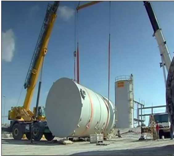
Above: Standing the tank vertically. They are using a third strap near the bottom to help pick up the tank vertically before raising the tank.
