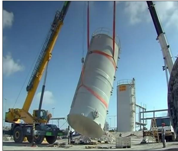
Above: Standing the tank vertically. They are using a third strap near the bottom to help pick up the tank vertically before raising the tank.
